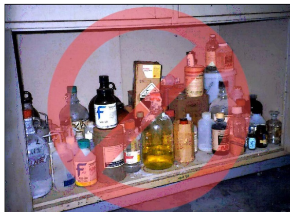
Figure VI-I. Improper Fume Hood Chemical Storage
